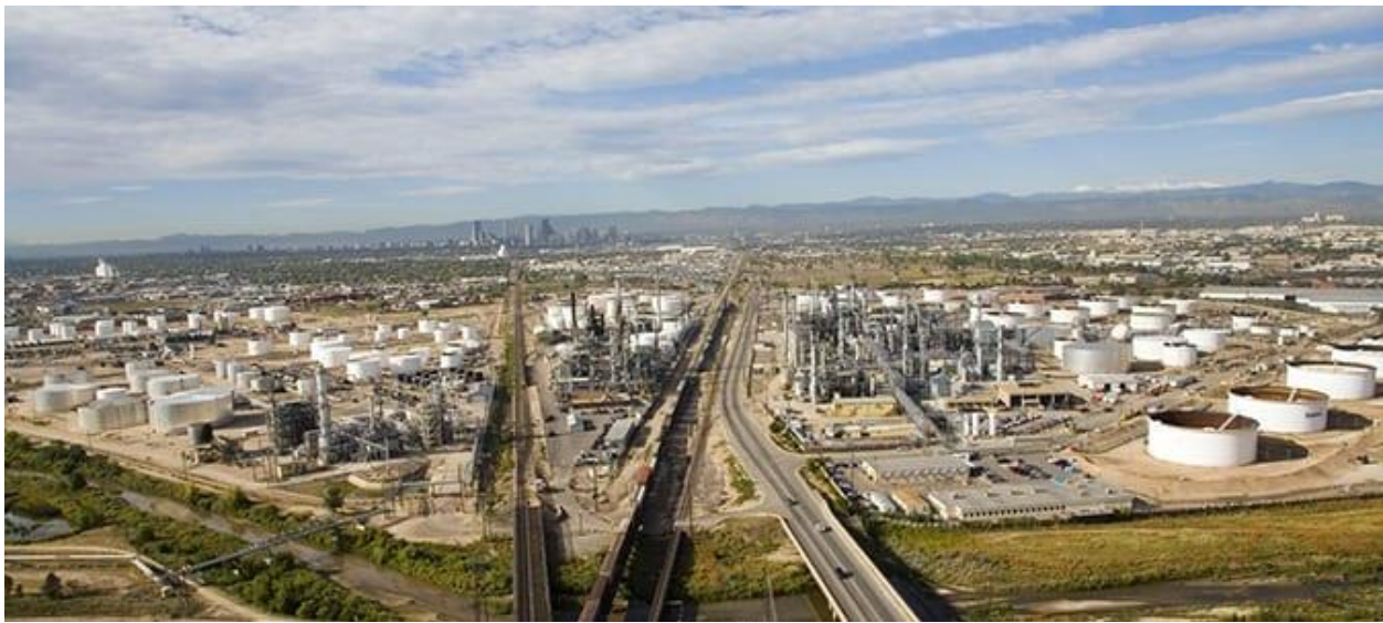
Suncor Refinery, Image at suncor.com
