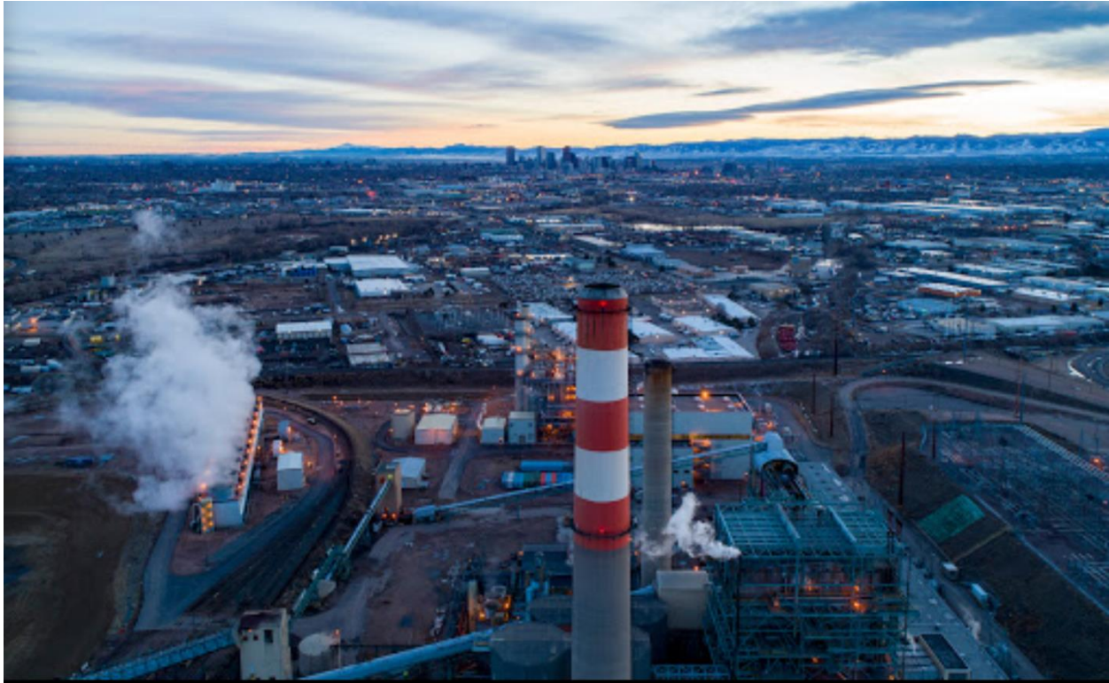
Cherokee Power Plant, photo by Gregor Tokarski 1/19
