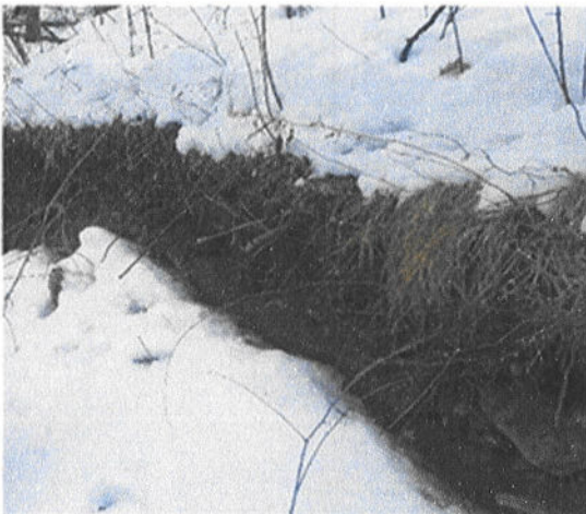
Rutting along road cut by logger to access timber on WWMA. This rut is approximately 4 feet tall and undercut due to erosion.
