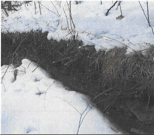
Rutting along road cut by logger to access timber on WWMA. This rut is approximately 4 feet tall and undercut due to erosion.
