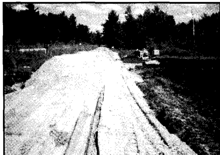
Step 3. The illegal placement of fill within the wetland completes the conversion to upland developable property.
