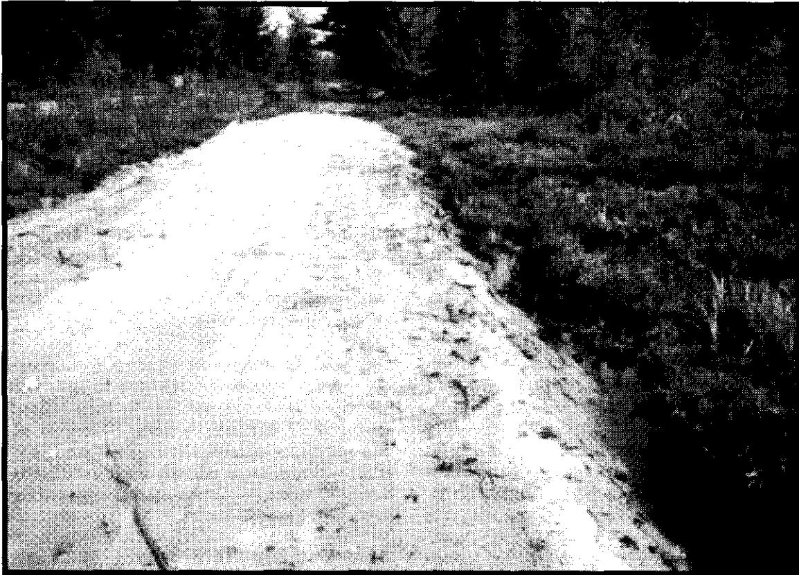
Illegal Access. Each year hundreds of unauthorized roads and driveways are constructed through Michigan's wetlands. Few of these violations are ever investigated by DEQ.
