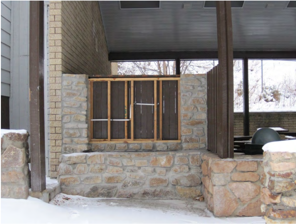
Figure 1 - Filling station under construction. Note proximity of table in adjacent concession food area
