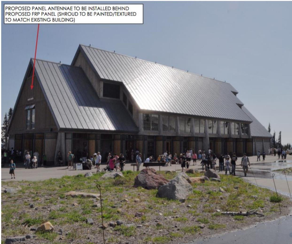
**Figure 3.** Jackson Visitor Center and location of proposed antennas on the interior of the east gable end. Antennas would not be visible from the outside.
