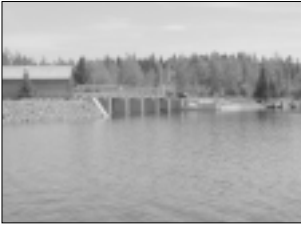
New and Improved! The State rebuilt Churchill Dam without permits.
