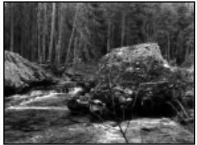
Man's Contribution: washed-out bridge at Chisolm Brook.
