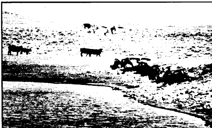
Use of car bodies to stop loss of front slope due to wave action. Montana.
